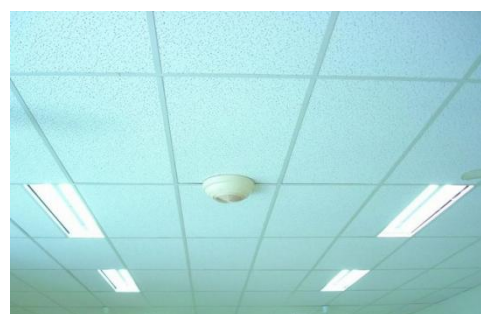
Typical suspended ceiling system
