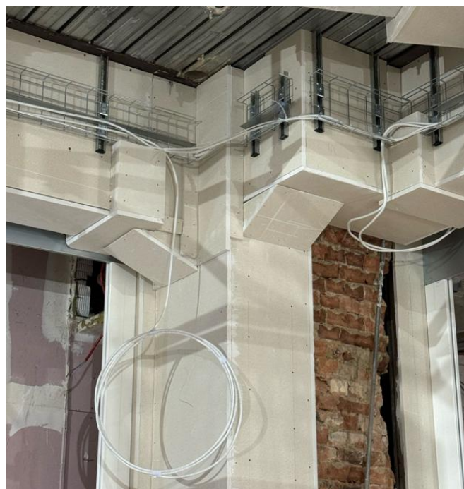
Board fire protection to steel
