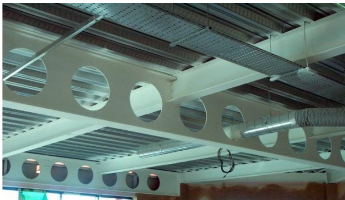
Intumescent (reactive) coating on cellular beams
