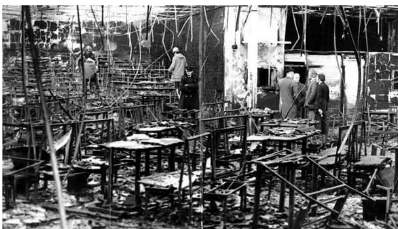
Flammable carpet tiles on walls of Stardust Disco Fire Dublin in 1981, in which 31 people lost their lives, contributed to fire spread.
