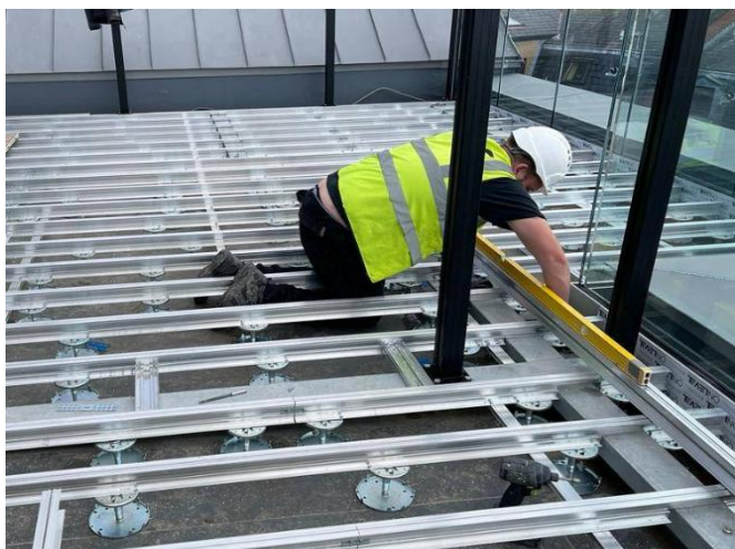
Installing a raised access floor
